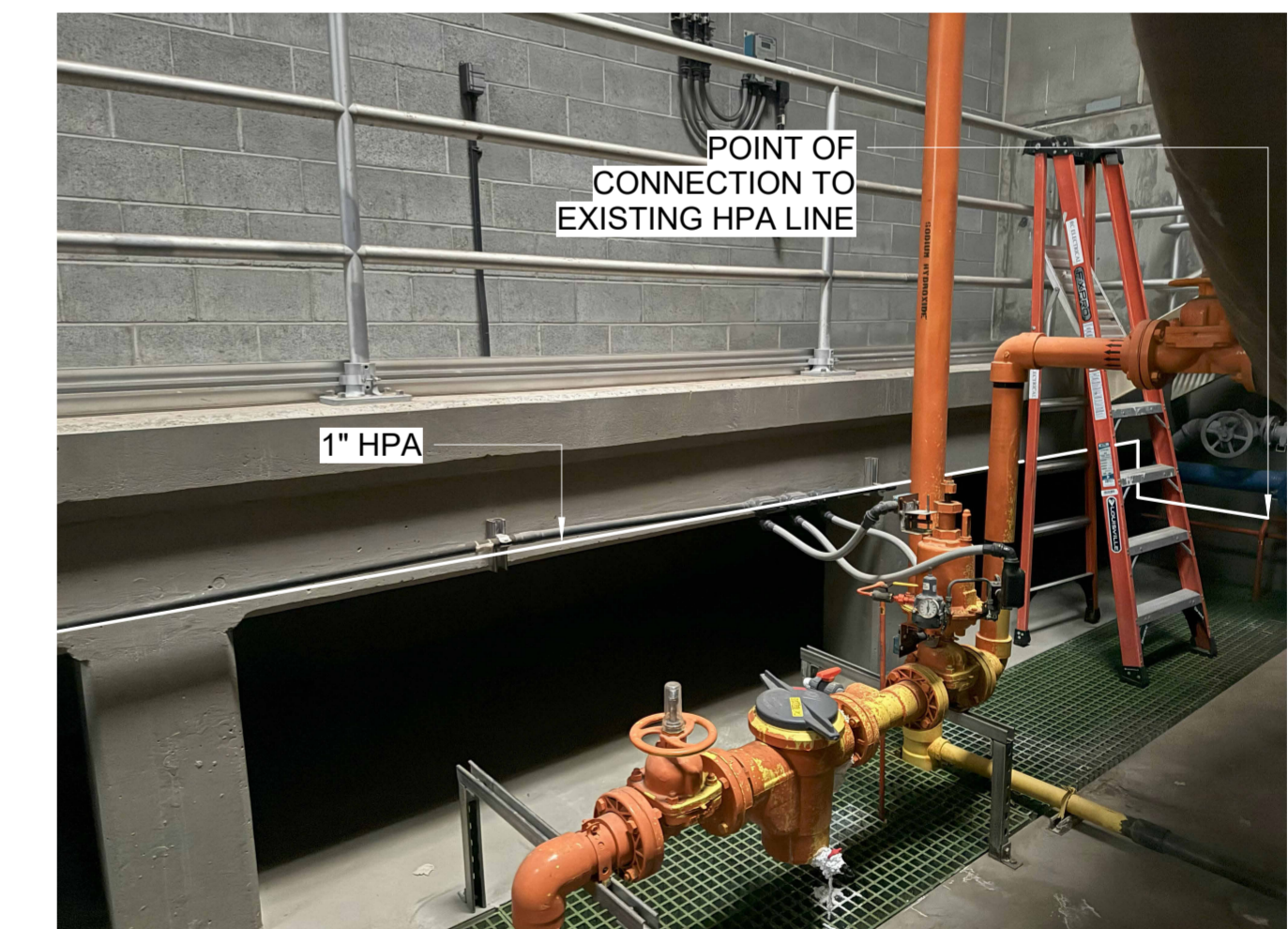
6 AIR LINE CONSTRUCTION CONNECTION NO SCALE
